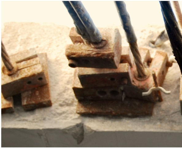
Photos: Bundled cables secured using single cable lock-off anchor that are stacked together.
