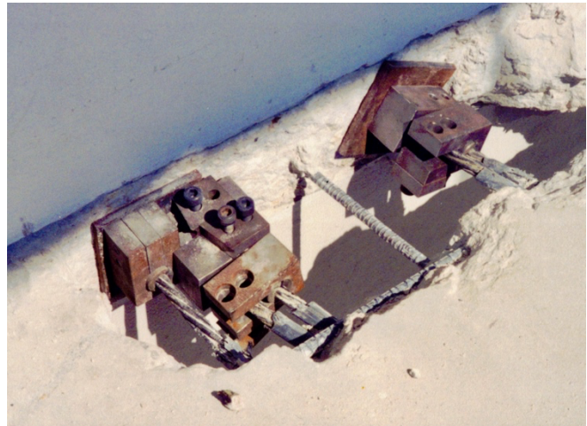
Photos: Bundled cables secured using single cable lock-off anchor that are stacked together.
